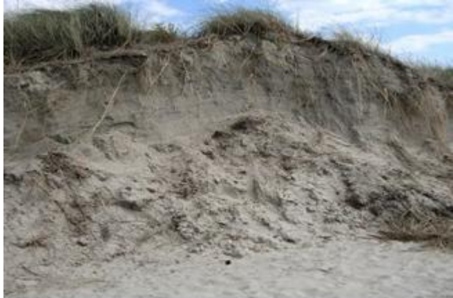
The dunal revegetation will be carried out over a length of 1.7 km on Kirra beach.
